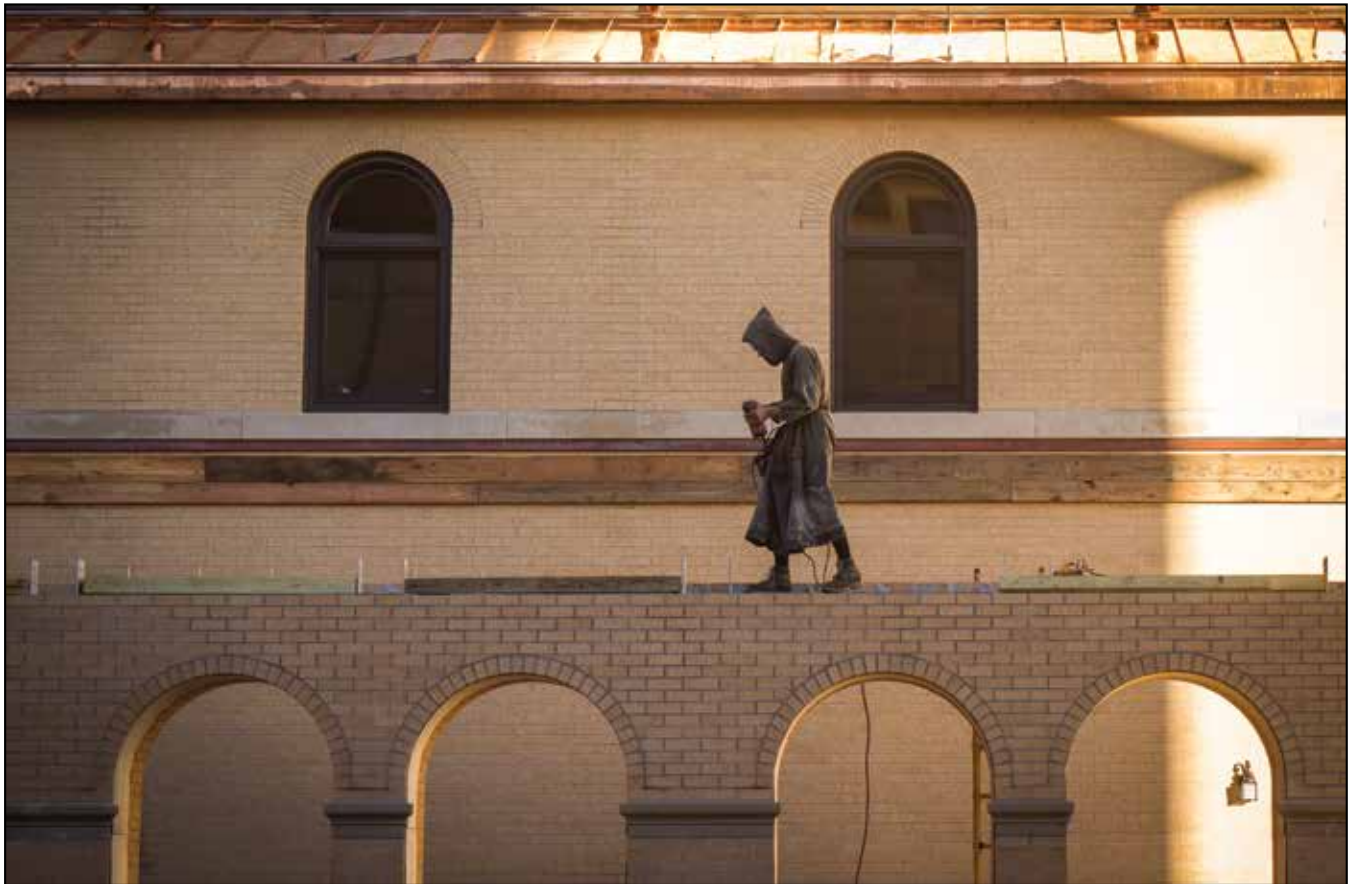
A monk prepares the cloister wall for a roof.
