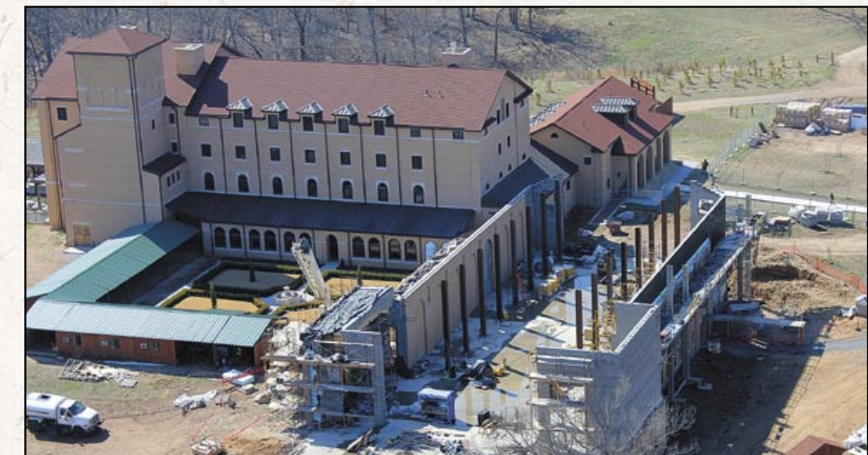
2011, March: Aerial view of construction of church
