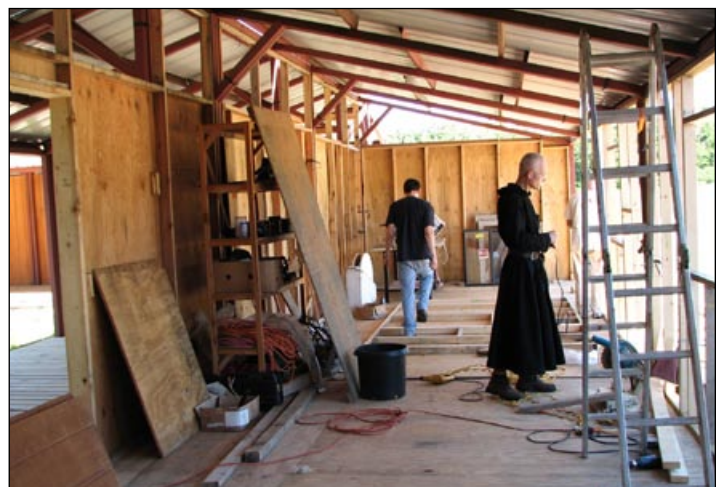
The beginning of the modular building.
