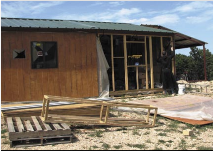
Modular building nearing completion.
